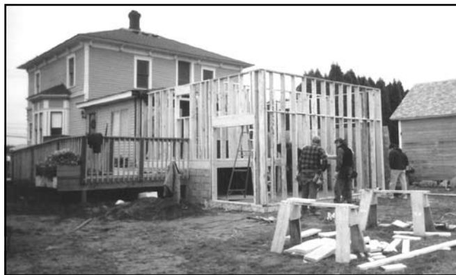
Construction on the Reiman-Simmons House.
