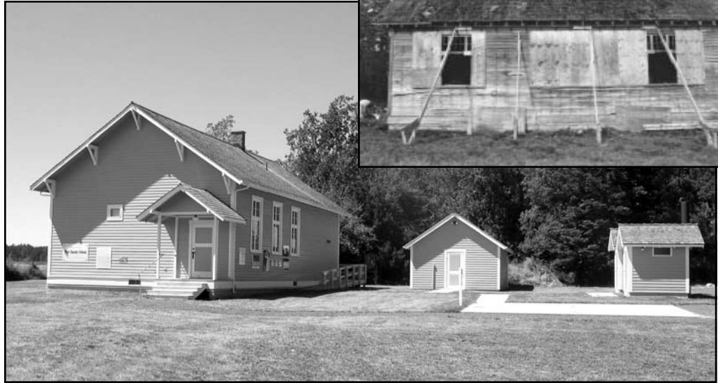
The Port Stanley School, before and after. Upper photo shows bracing added for snow load.
